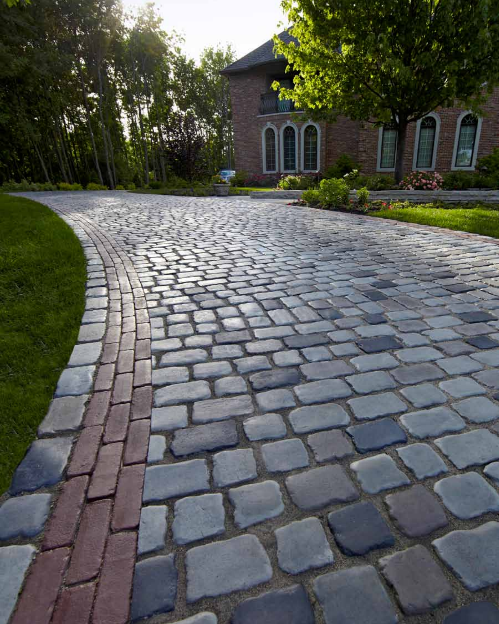
Pavers - Courtstone® (Basalt, Belgian Blue and Dawn Mist, blended on site) with Copthorne® accent.
